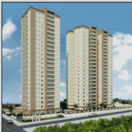
SALETE RESIDENCES CLUB ORBAN RUA SALETE, 279 – SANTANA – SÃO PAULO A= 29.000M 2 / CONCRETO ARMADO
